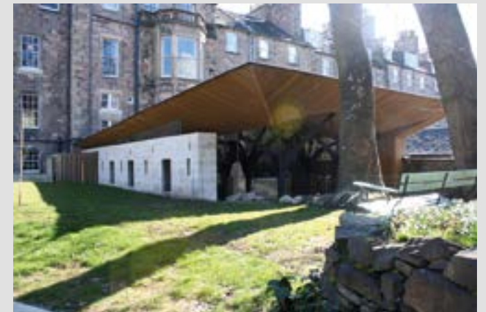
Frameless glazing—George Square Lane Glazing is used to create the effect of a floating roof on this building.
