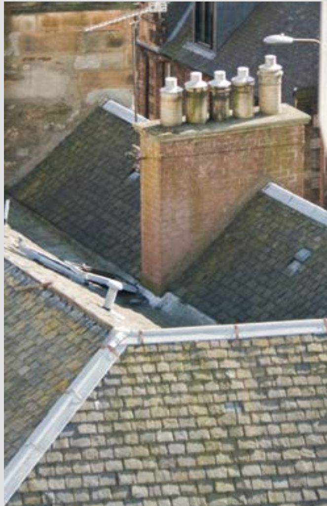
Traditional roofing materials (right) Slate, Lead and zinc are traditional roofing materials used in Edinburgh—seen here from the Museum of Scotland’s roof.
