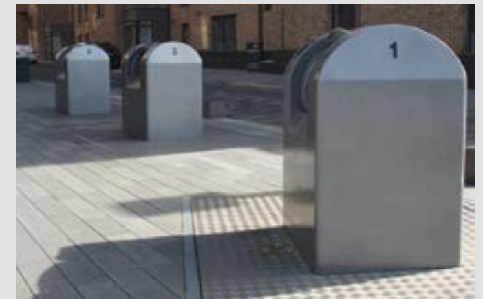
Underground bins for residual waste allow large volumes to be held with minimal impact on the street scene. It is important that the Council's Waste and Cleansing Service are involved early, as their requirements may impact on the design.
