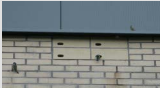
Swift Bricks—Beaverbank Place On this development in North Edinburgh swift bricks have been designed into the external wall. These should be shown on planning drawings.
