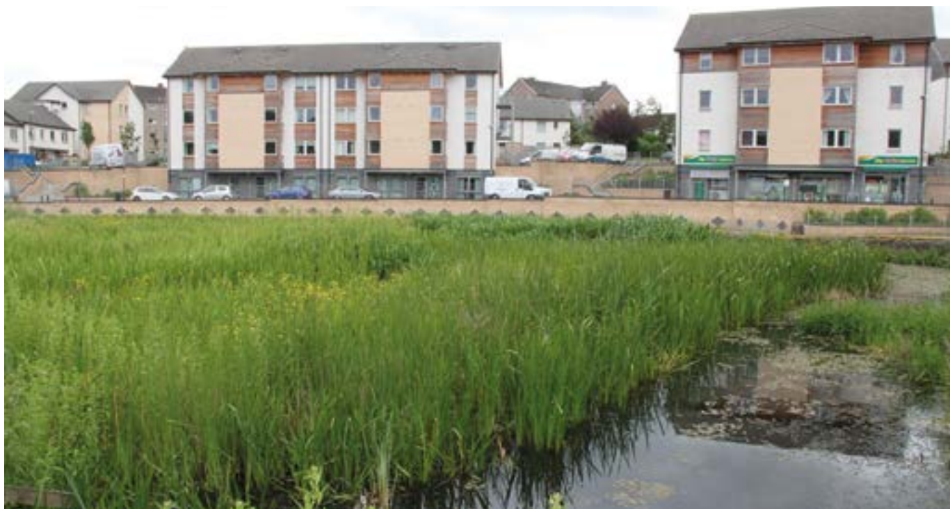
SUDS retention basin, Firrhill Neuk, Oxfangs
