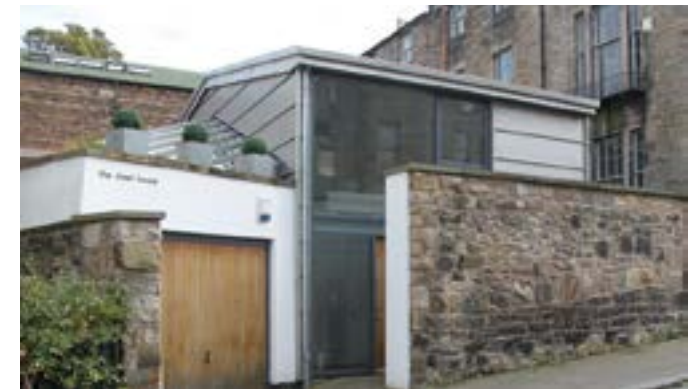
Incorporating a boundary wall—Hart Street This stone wall was re-used and incorporated into the new house.
