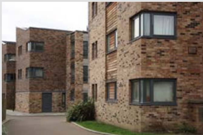
Subtle variation—Telford March Two different mixes of brick have been used to provide variation in colour within the elevations.
